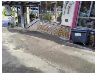
External path from main to side entrance
