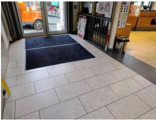
Path from the side entrance to the cash desk
