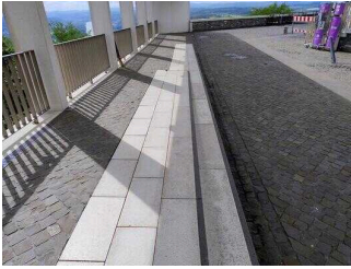
Ramp to the entry of the mountain station
