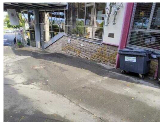
External path from main to side entrance ©Randolph French
