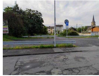
Parking lot next to the railway track
