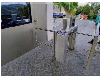
Mountain station entrance
