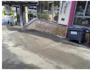
External path from main to side entrance
