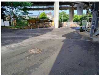
External path from main to side entrance
